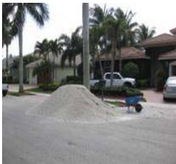
\frac{3}{4} " to \frac{1}{4} " Primary Base Drain Rock
