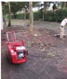
Sod Cutter Removal
